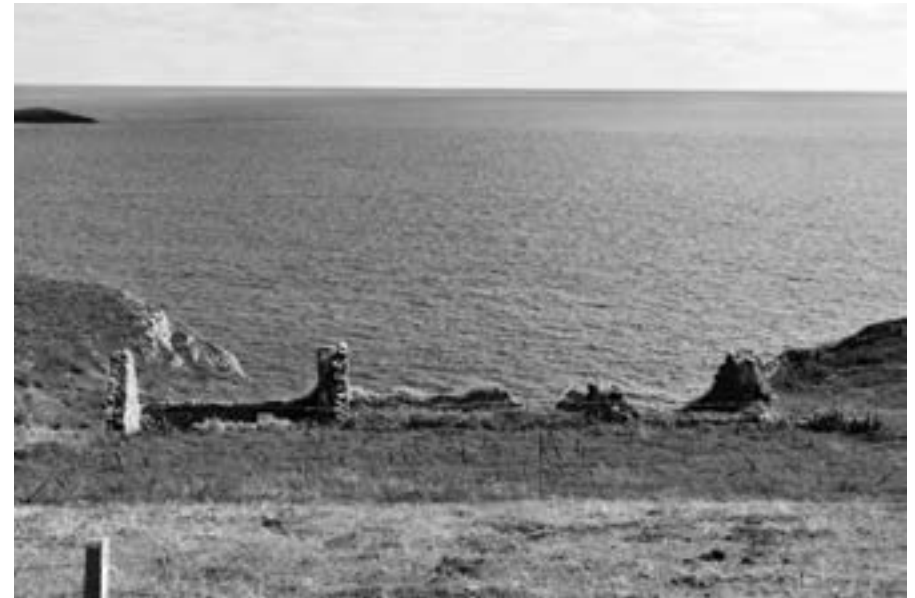
Fig. 3: The ruins of the home of David and James Brickley, in the townland of Lehenagh, Co. Cork, who died on board HMS Defence in the Battle of Jutland. The house became ruinous after a house fire in the 1950s (Photo: author 2013).
